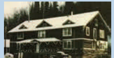
Chase-Chapman Building, Anvik
